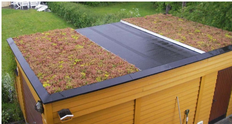
Figure 7. The roof with the three sections.
