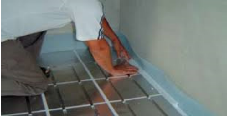
Figure 2 Installation of Comfort floor system
