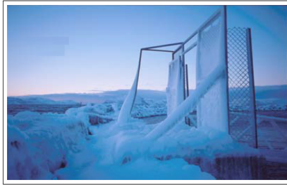
Figure 11.14: Icing of facilities at Melkøya during winter 2002. Source: M. A. Drage et al. 2003 [59]
