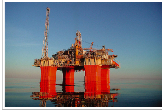
Figure 4.5: Semi-submersible platform at Snorre field in the North Sea. Source: Oil Rig Photos
