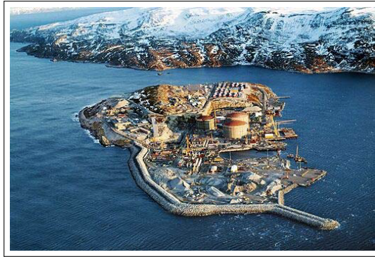
Figure 9.10: Icelandic type berm breakwater protecting Melkøya terminal, Norway. Source: Statoil
