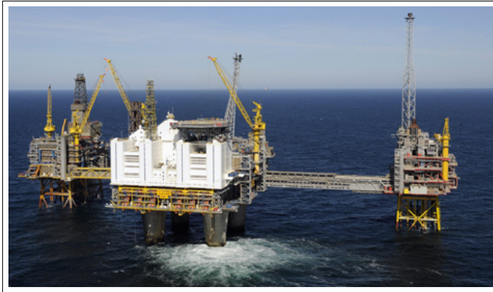
Figure 4.3: Concrete based and steel jacket platforms in the Oseberg field in the North Sea. Source: Statoil
