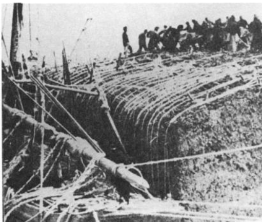
Bilde 1 «Repairing scene of a broken dyke with bamboo and timber in China in 1935» (YAMANOUCI, T., 1986)
