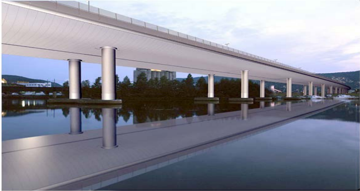
Figure 6.4 The old and the new bridge side by side after the pier of the old bridge upgraded to a circular cross section (after Grete Trevdt)
