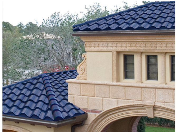
Fig. 3. Curved clay looking solar tiles [55].
