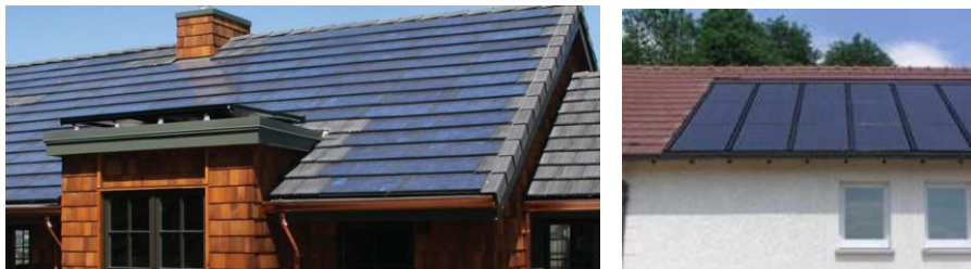
Figure 1. Examples of BIPV tiles (left) and BIPV modules (right) (Applied Solar 2010 [4], DuPont 2011 [5]).
