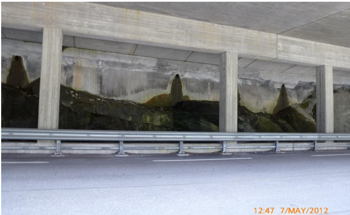
Figur 6-49 Ramsteina – Drenering under overbygget
