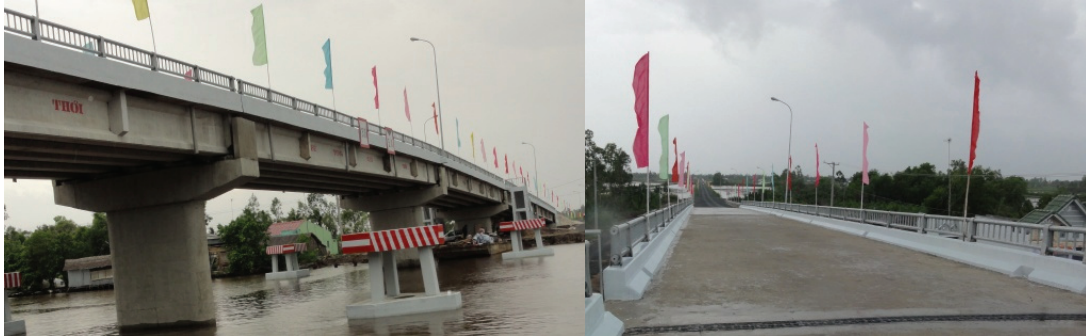
Figure 9: U Minh Bridge, August 2011
