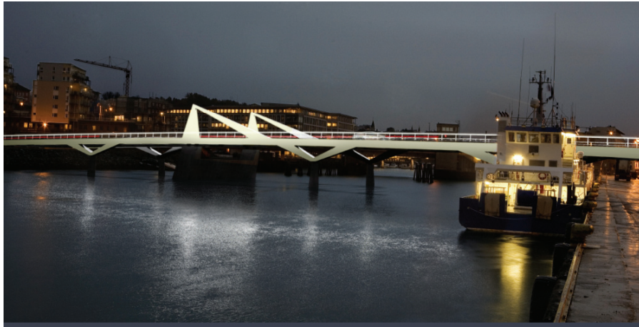
Figure 14: River Nid Bridge
