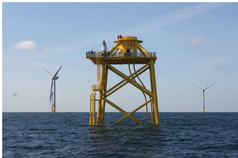
Figure 7: Truss structure for support of wind turbines (Tørum, 2011)
