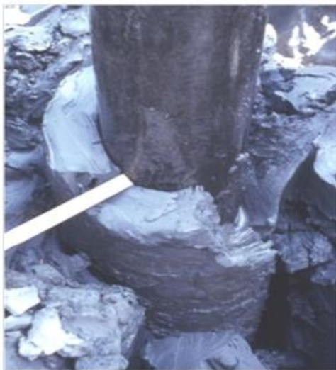
Figure 2.2.17- Picture from extraction of pile A10 out of the ground, Haga (after Karlsrud and Haugen, 1984).
