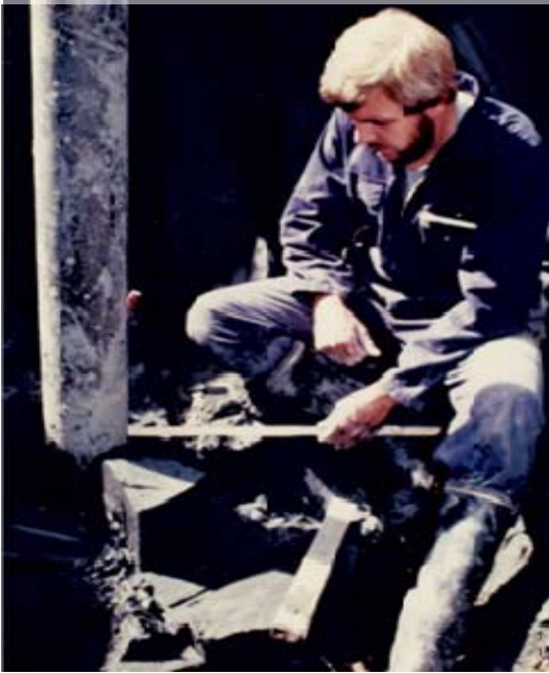
Figure 2.2.16- Picture from trenching and block sampling next to Pile A10, Haga (after Karlsrud and Haugen, 1984)
