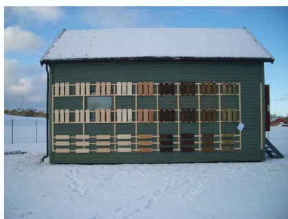
Figure 1 Test house, eastern facade (feb 2005)
