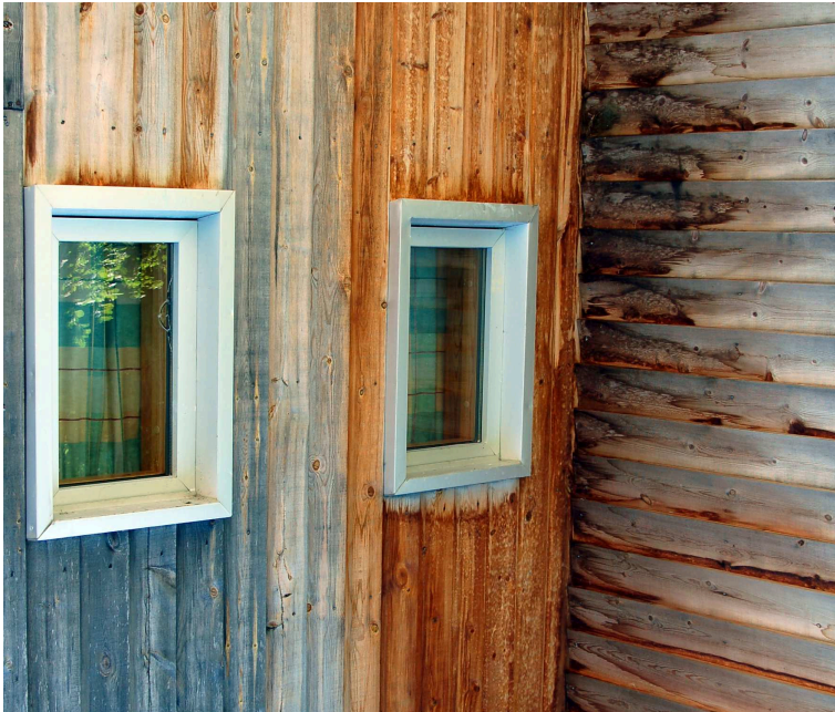
Figure 6.3.: Different colors of aspen cladding, Tyholt crematory, Trondheim, Norway
