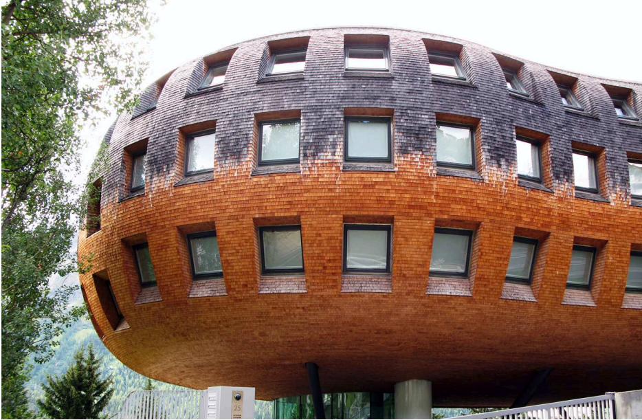
Figure 1.1.: Wooden shingle cladding at Chesa Futura by Norman Foster in St.Moritz, Switzerland, photo Claudio Castellacci
