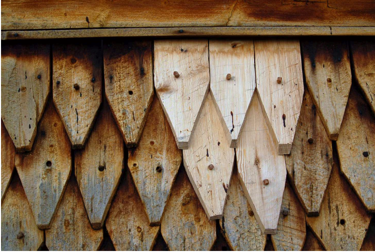
Figure 3.1.: Wooden shingles, facade detail from Eidsborg stave church, built in the 13 th century.
