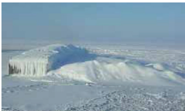
Figure 2.5.1 Grounded barge in the NCS, with spray-ice added to increase sliding resistance (Bastian et al., 2004).
