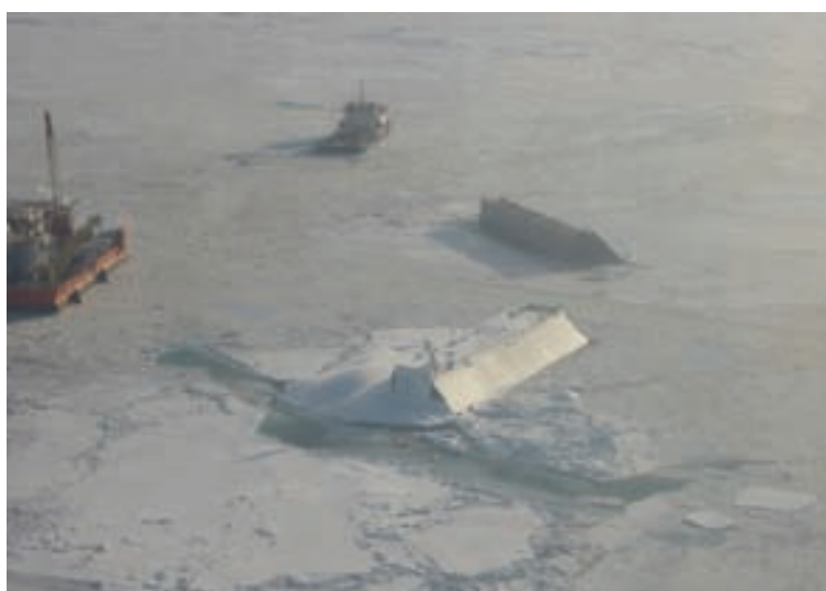
Figure 2.5.2 Purpose-built ice protection structure in the NCS (Courtesy of IMPaC).
