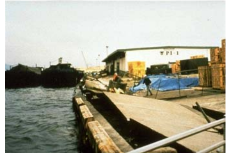
Retaining wall damage and lateral spreading Kobe, Japan, 1995
