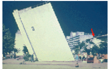
Retaining wall damage and lateral spreading Kobe, Japan, 1995
