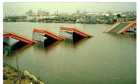
Collapsed bridge, Niigata, Japan, 1964
