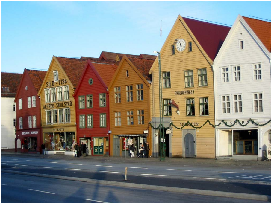
Figure 9.4: Bryggen in Bergen 1995, divided from the sea-front by a busy four-lane main street.
