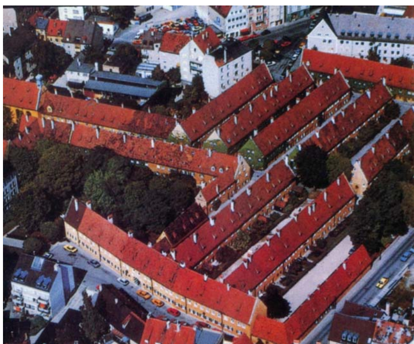
Figure 3.2: Fuggerei in Augsburg (1516-23), an attempt to realize the utopia by Thomas More, erected in the early 15 th century to house retired weavers and the deprived. It was severely damaged during World War II.
