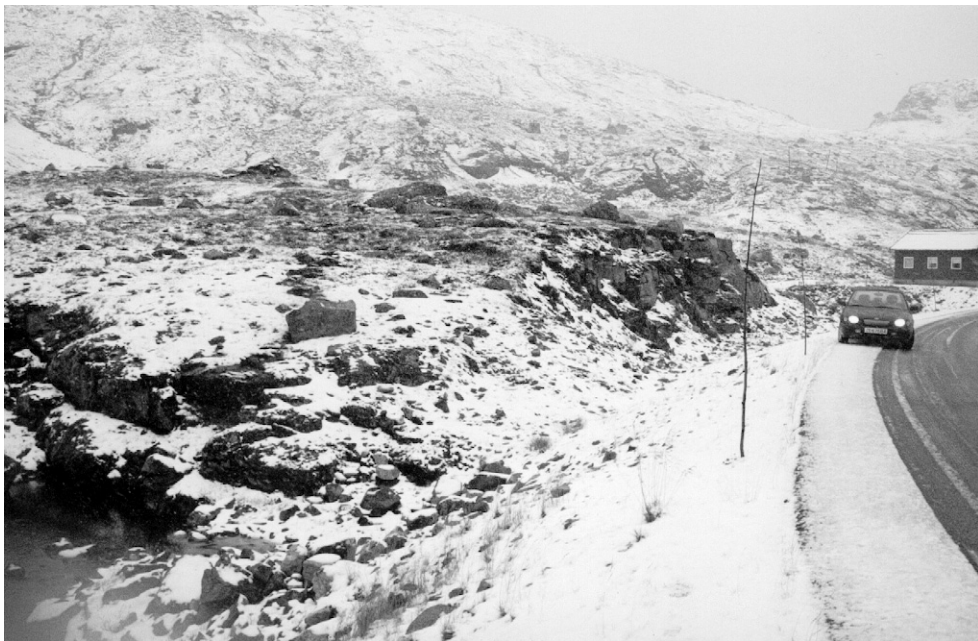
Figure 6.14 Troublesome cut section at location “A” (Figure 6.13) in Kaperdalen.
