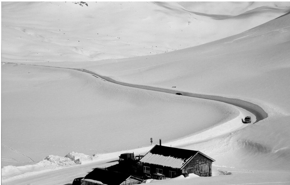
Figure 6.12 Photograph taken in April 1999 in Kaperdalen. The caravan to the right is passing profile 4020. The high snowbanks along the road increase the vulnerability of the road to snow drifting.
