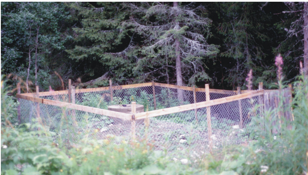
Figure 5.3.1 Example of fencing (approximately 20 m 2 ) around a groundwater well in bedrock. The size and design of the fences varies between the waterworks in Dataset E mod .
