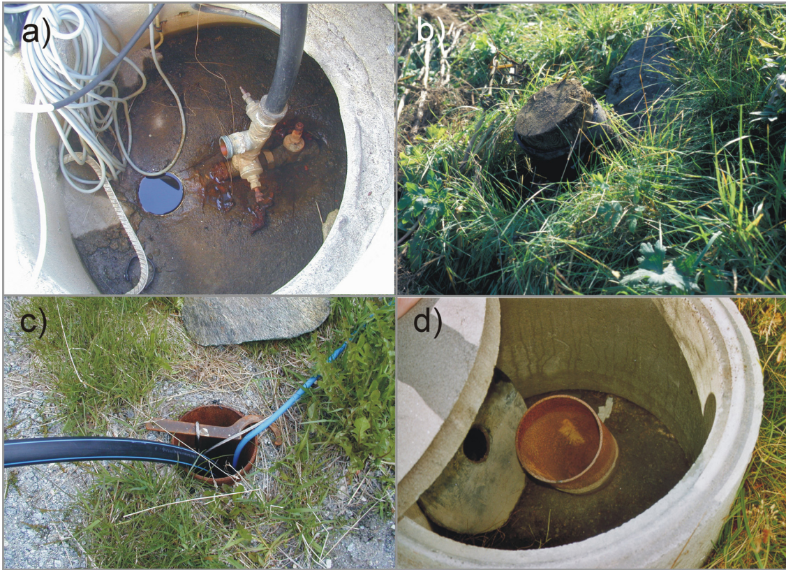
Figure 5.3.10 Typical examples of abandoned wells (Pictures a and b) and wells not yet in use as supply wells (Pictures c and d).
