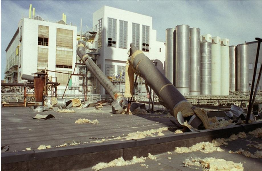
Figure 1.1: A view of the pipeline that was destroyed during the incident at Hydro Agri Porsgrunn (Norsk Hydro ASA).
