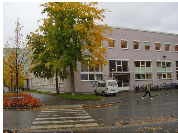
Figure 5.3. The west facade
