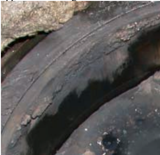
Figure 3-45 Severe flame ring deposits.
