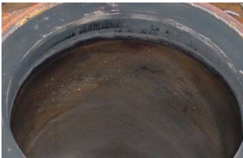
Figure 4-37 Picture of the liner at inspection one
