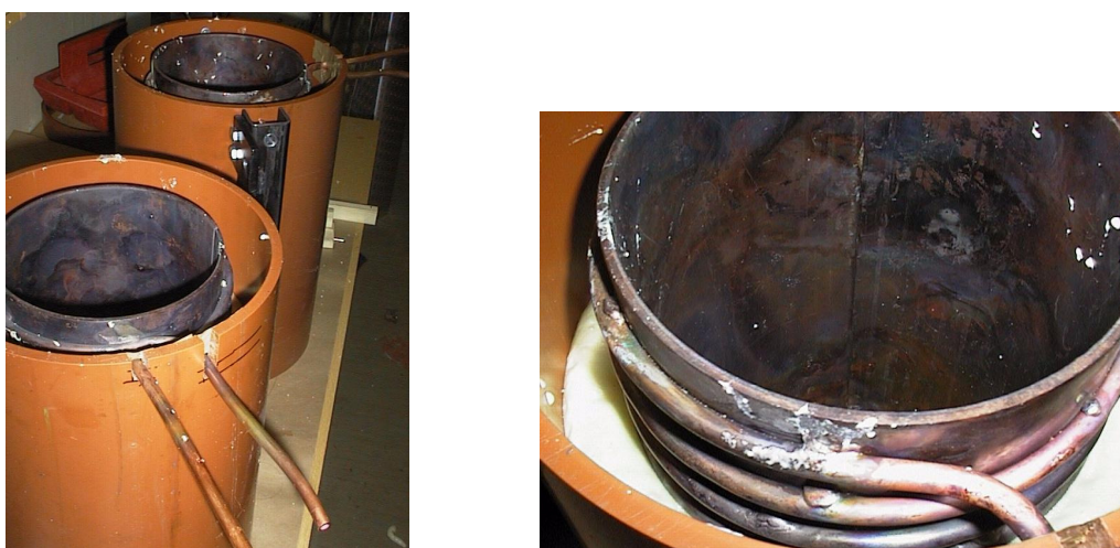
Figure 4.9 Temperature control chambers under construction, consisting of 5 mm copper-cylinder, water copper tubes and plastic mould.
