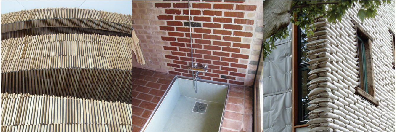
Figure 8: Physical properties of building components can meet constructional and environmental challenges, and at the same time substantiate tectonic relationships.
