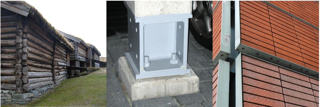
Figure 5: Reversible connections can take a variety of shapes, and joints are often refined sections of the architecture in both vernacular and modern designs.
