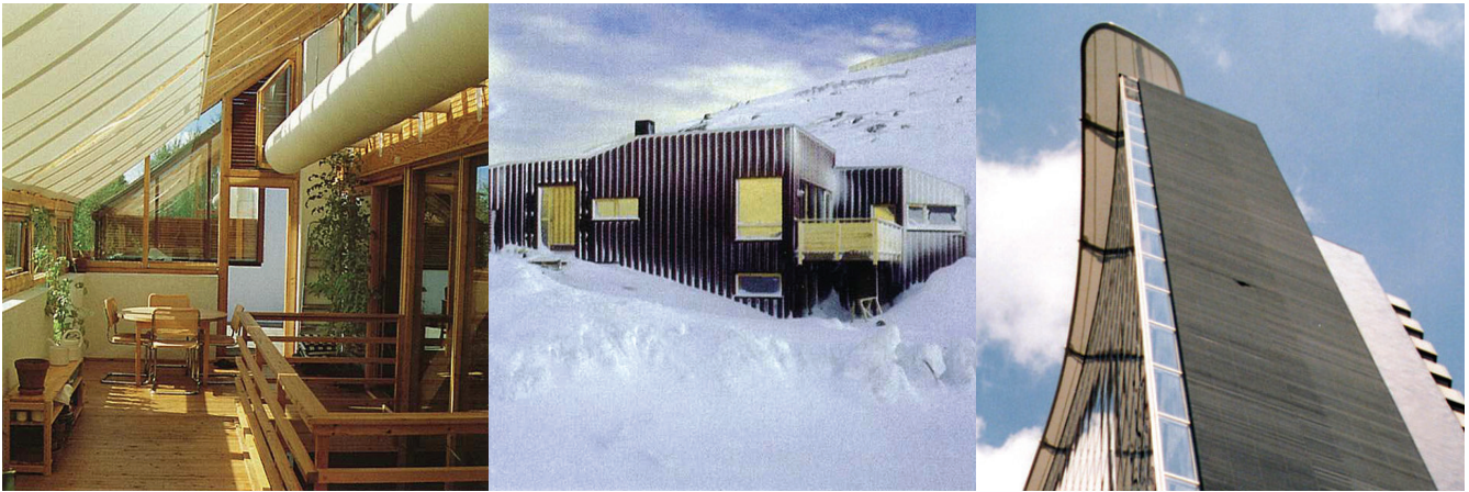
a) Norway: Sunroom in passive solar dwelling, Trondheim. Architect: Sintef/ Hestnes 1982. (Photo: F. Østmo) b) Norway: Wind adapted dwelling reduces snow drifts in Hammerfest. Architect: Børve/ Bjørge 1989 (Photo: O. B. Hansen) c) Germany: Wind roof facilitating natural ventilation at GSW Headquarters, Berlin. Architect: Sauerbruch Hutton Architects 1999 (Photo: T. Kleiven)
