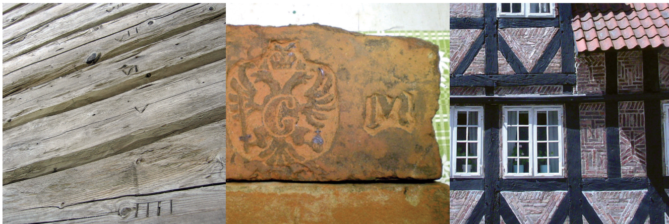
Figure 7: Useful information regarding salvageability can be carried along with the components as well as along with the architectural language
