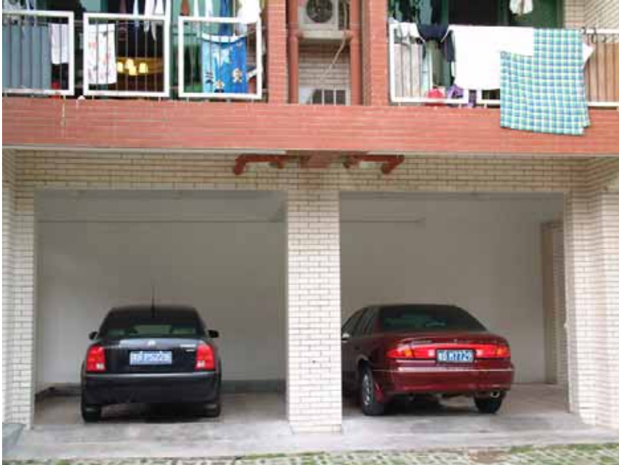
FIGURE 7.8 Parking lots on the ground floor of a housing building in Meilin Yicun Housing District
