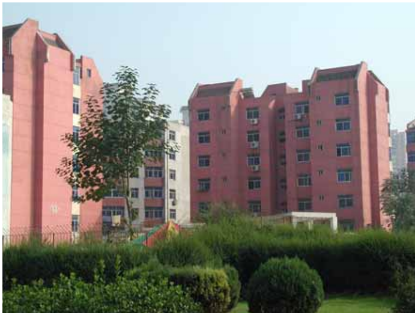
FIGURE 6.4 Anju Project housing in Ming De Men Housing District
