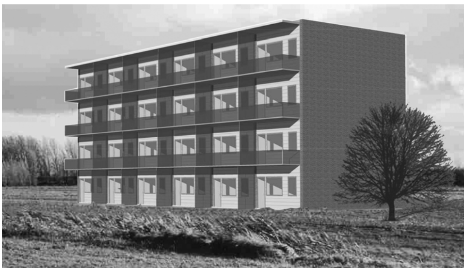
Figure 1 The dwelling model is a four storey apartment building with 24 flats
