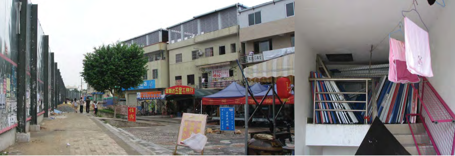
5.36b Rooftop units in Nanting Cun accessed through hole in the ceiling. Author's photographs, 2011.
