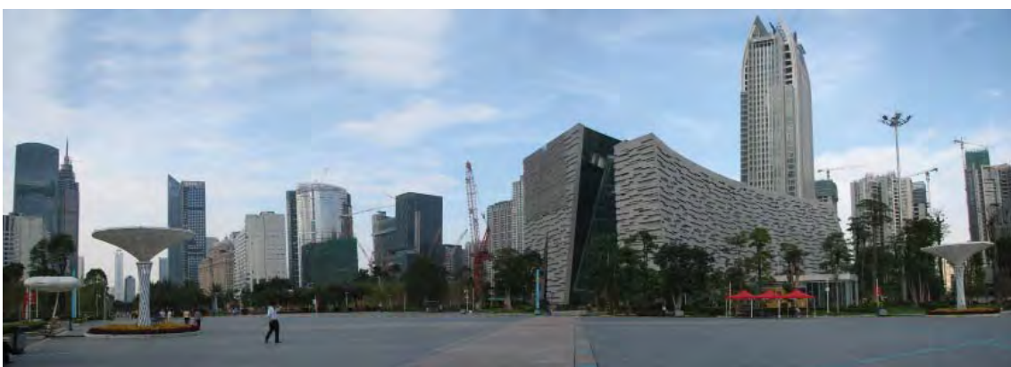
2.11 Old and new main library. Author's photographs, 2011.
