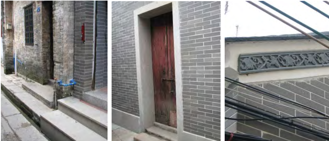
5.33a Redecorating old houses in Xiaozhou Cun. Author's photographs, 2011.
