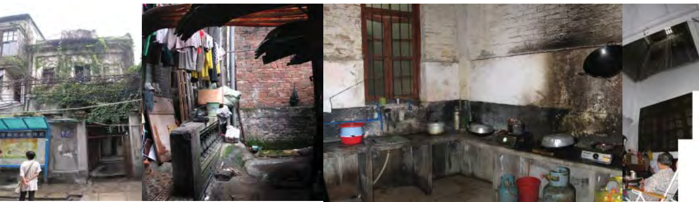
5.38a Old dwelling house. Author's photographs. 2011
