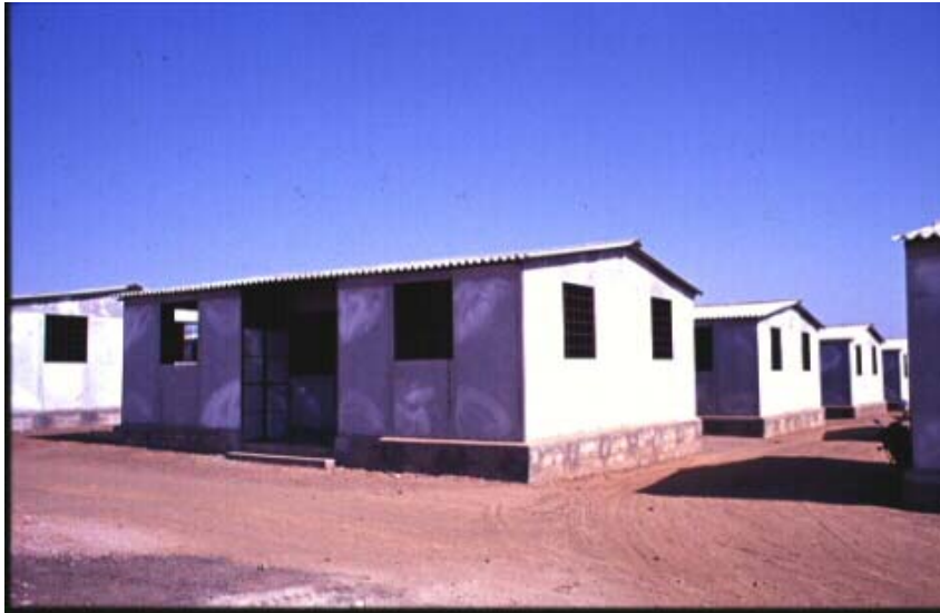
Fig. 8.20 Expensive temporary shelters in cement sheets and metal frames made by Indian Oil Corporation Sep. 2001
