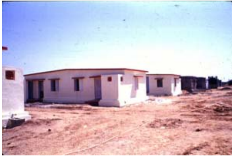
Fig. 8.28 Permanent housing reconstruction in concrete blocks – ‘Adopted’ village Chandrani in Kutch Oct. 2001
