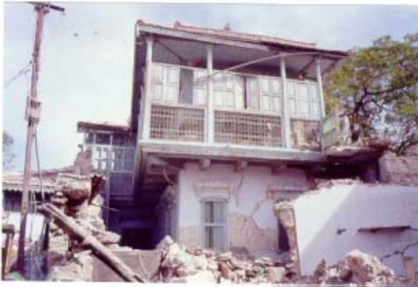
Fig. 8.16 Surviving balconied house in wood and masonry in Anjar after 2001 earthquake Feb. 2001
