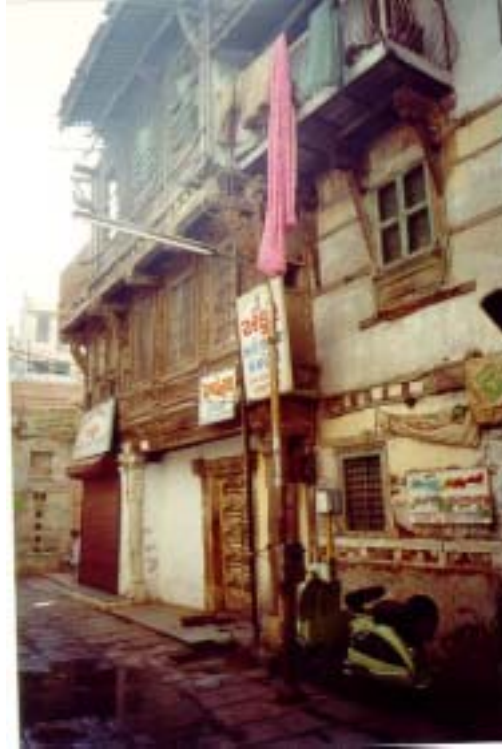
Fig. 8.12 Timber laced housing in Old Ahmedabad also performed remarkably well in 2001 earthquake
