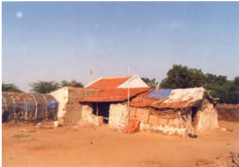
Fig. 8.24 Permanent, semi-permanent and temporary structures get added to make one house Sep. 2001
