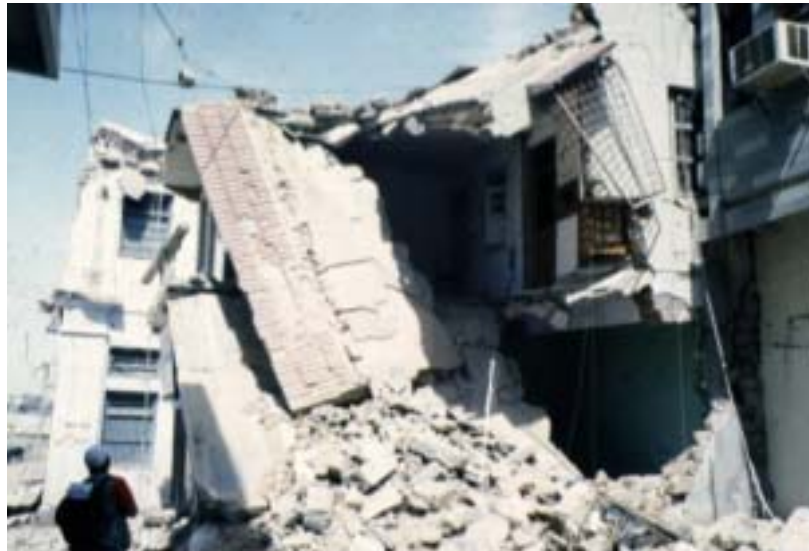
Fig. 8.14 Poor modern construction fell like pack of cards Feb. 2001
