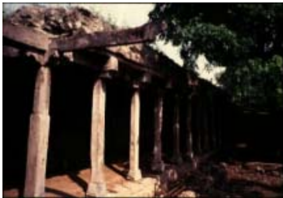
Fig. 7.5 Traditional Malwad Construction
