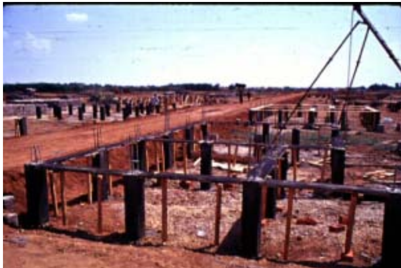
Fig. 8.29 Pile foundation of permanent reconstructed houses in village Chandrani Oct.2001
