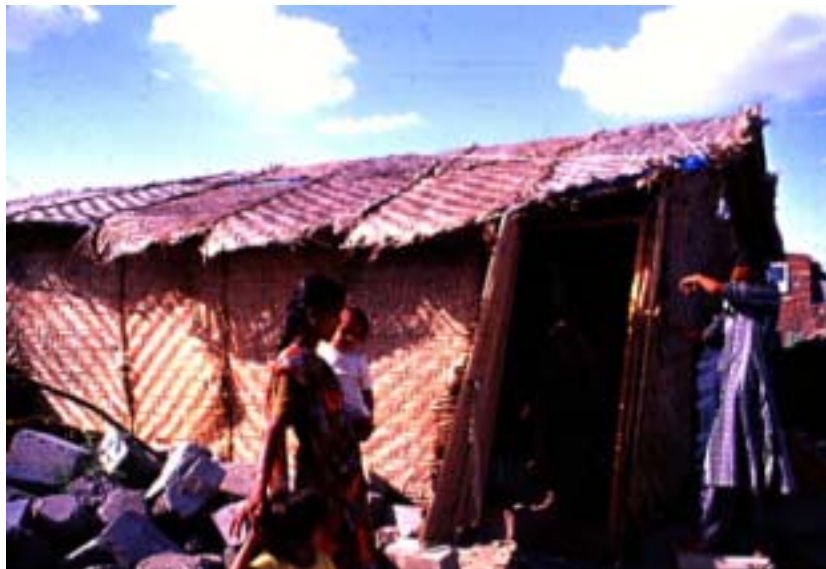
Fig. 8.19 Temporary shelter in Bamboo and Chatai provided by an international donor agency in Bhachao Sep. 2001
