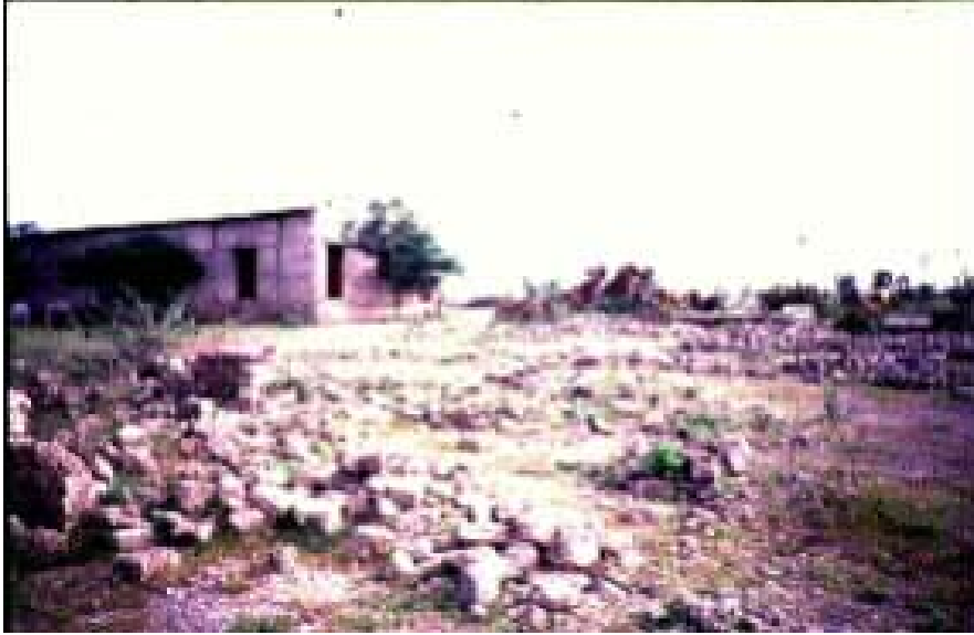
Fig. 7.19 Building centre lying vacated with unused concrete blocks
