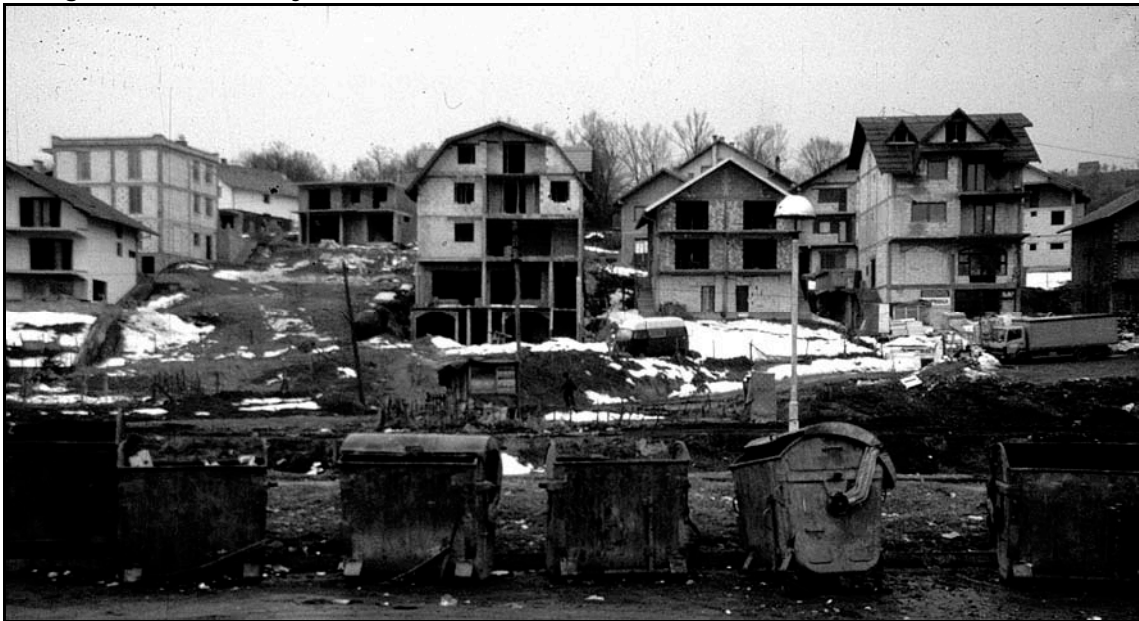
Fig. 6.2.6 Half-Finished Houses of today. They are somewhat similar to some of those completed by NRC during the latter part of the war, although those shown are larger than most of those included in the NRC scheme.
