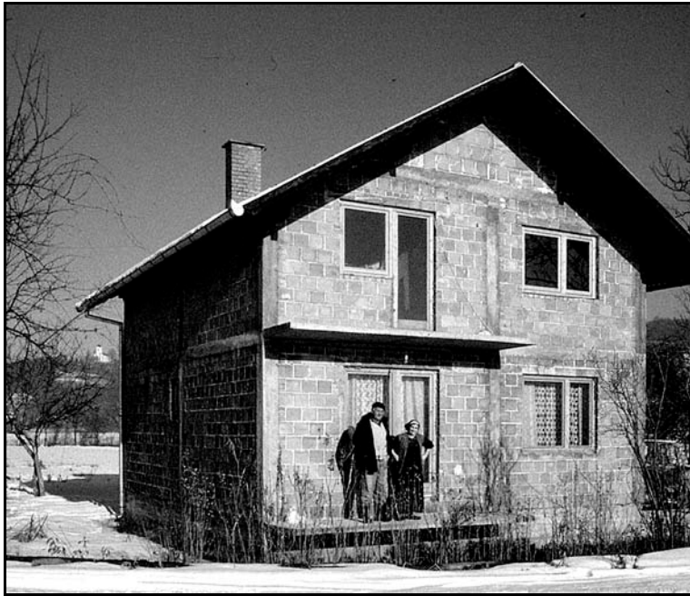
Fig. 6.5.23 The house rebuilt, January 2002, after it was totally demolished by artillery fire on May 10 1992. The efforts and sacrifices brought into its reconstruction signify its extraordinary ontological value.
