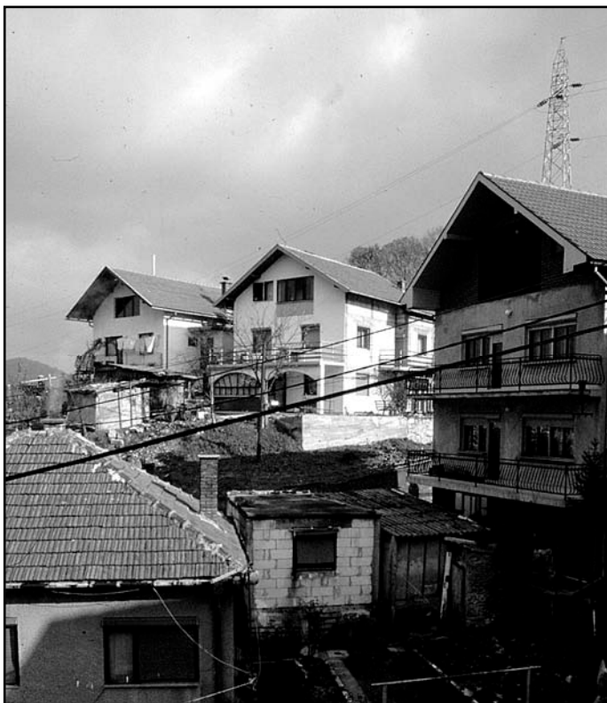
Fig.6.3.1 A central quality in the NRC Model was the location of the houses. Most of them were centrally located which meant that services and infra-structure was already in place and no major such investments were required. The children went to the local schools.
