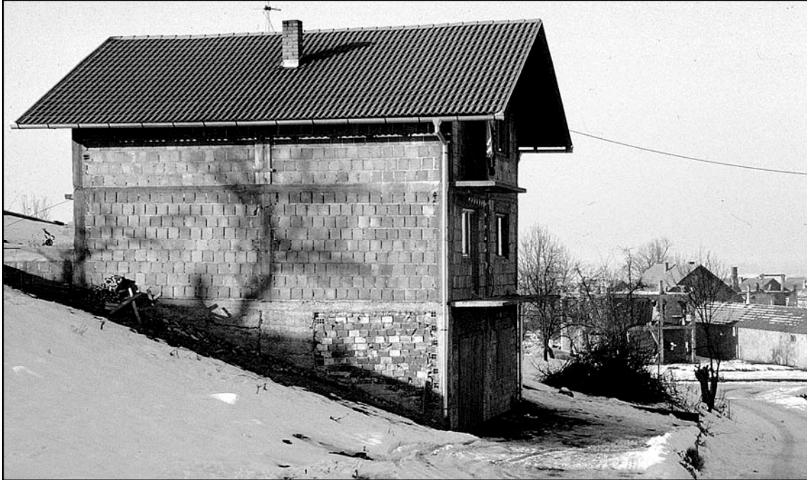
Fig.6.5.14 This is one of the houses extended beyond what the SRSA materials made possible. This was achieved with some extra financial input, with the use of recycled materials, and by the owner doing most of the work (The walls reveal different levels of professional capabilities as well as different sources of materials).
