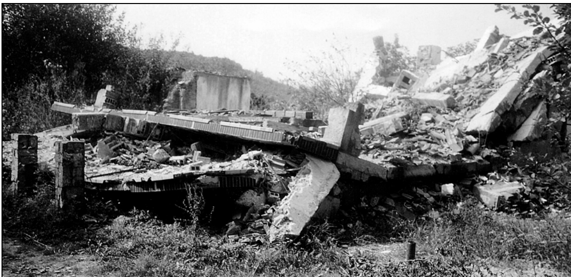
Fig. 6.5.8 The upper picture shows Hamid Spreco's House in Grapska in the Summer of 1999 as they were clearing the site for reconstruction and return. The house had been torched and sought destroyed by smashing the walls. The roof timber was most probably dismantled and re-used on some other house or sold. The lower picture shows the house after it was dynamited in August 1999 a mere week before the first UNHCR organized return visit. Having stayed abroad during the war Hamid Spreco did not qualify for SRSA support. Doing a full reconstruction from private funds alone was beyond his means. He was still in displacement looking for donors during my last visit in the Spring of 2001.
