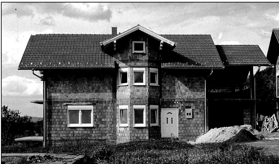
Fig. 6.5.17 A house financed in total from money transferred from a Grapska family living and working in Norway. Most of the materials used are brought in from abroad. Note the imported PVC coated window frames mounted partly to reduce annual maintenance for the owner living abroad. Such un-Bosnian features tends to raise the perceived status of the building, cf. the failed slogan of the Bosnian tile factory referred to on page 197.
