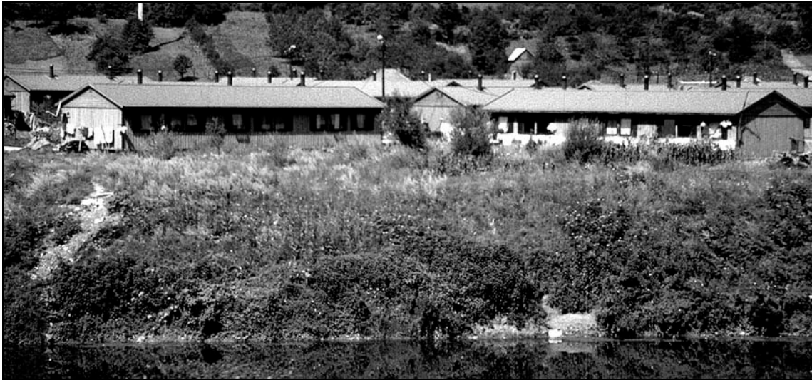
Fig. 6.4.1 Norwegian prefabs erected by the industrial sites of Zenica. One of NPA's first building projects in Bosnia-Herzegovina.
