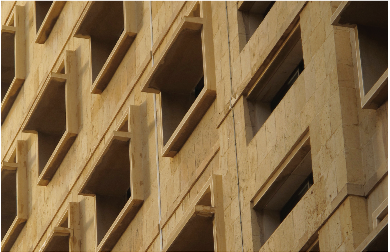
Sun shading integrated in the concrete facades.
