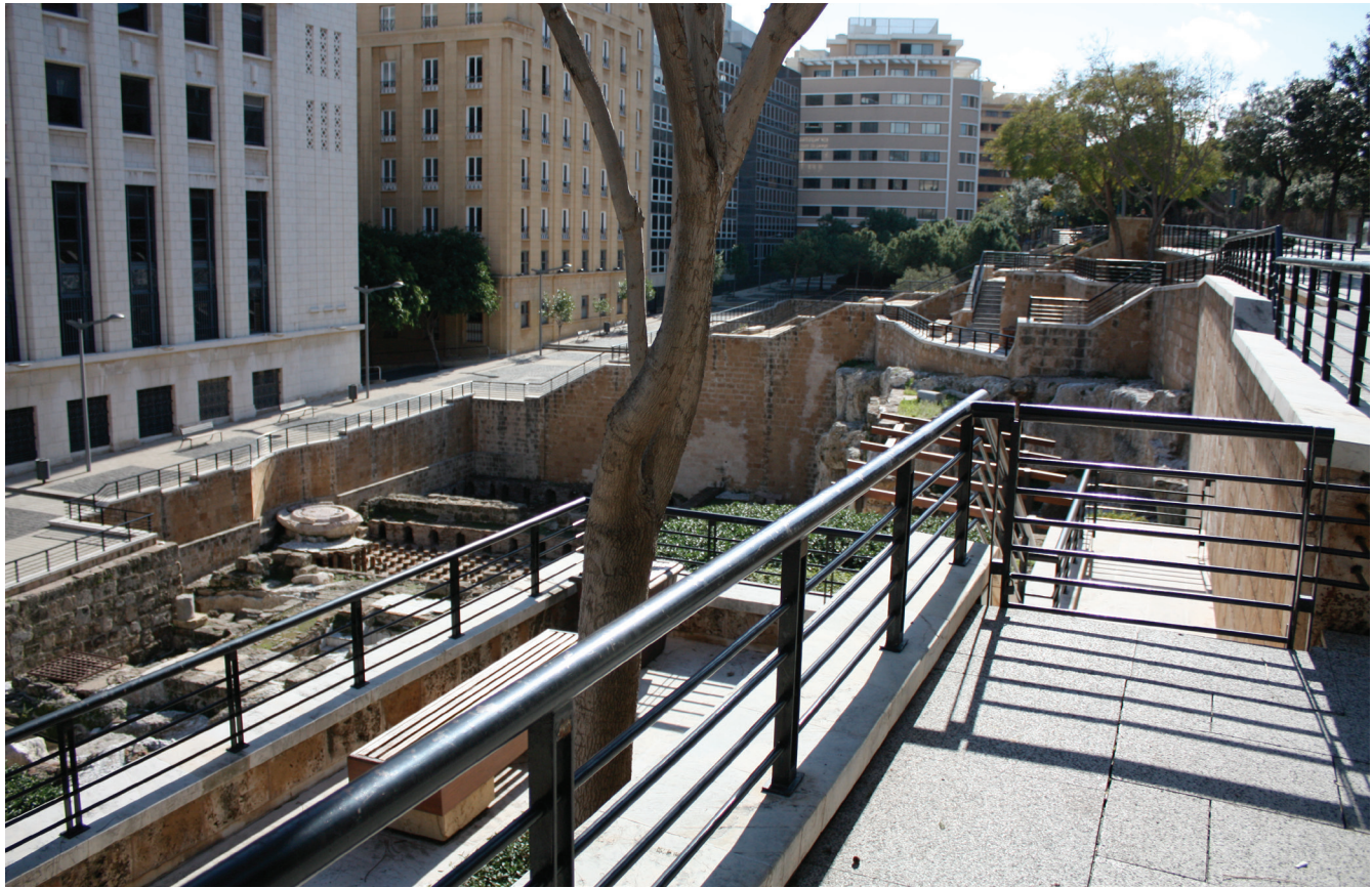
The Roman Baths located on the eastern slope of Serail Hill. The scene consists of ruins originally discovered in 1968-69, but developed as a public space in 1995-97. Being a public space it is rather odd that the plateaus are closed off with fences and trespassing is not allowed.
