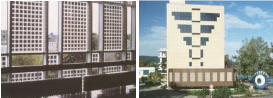
Figure 2-13. Left: Crystalline silicon PV cells between glass panes in a German building (Pilkington Solar AG). Right: PV modules as a patchwork on a building in Switzerland (Solution AG).
