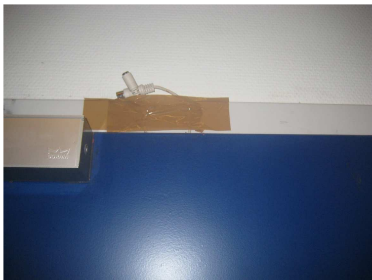
Figure 1: Gaining access by a short cable and tape
